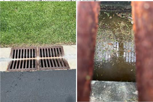
**S-66:** Contains 8-10" of sediment in sump of structure.
