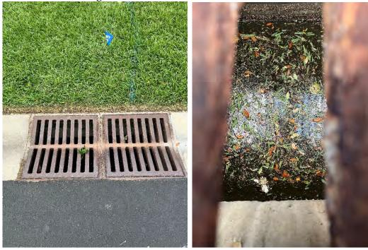
**S-60:** Contains 6-8" of sediment in sump of structure.
