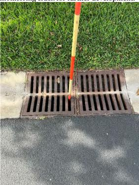
**S-30:** 6-8" of sediment in sump of structure. Also the curb is cracked at the west side of VGI.
