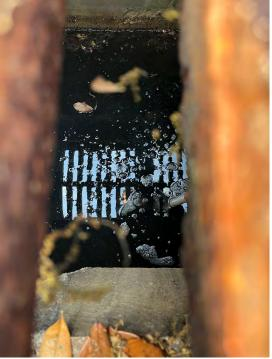
**S-52:** Contains 6-8" of sediment in sump of structure.
