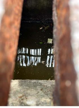
**S-57:** Contains 6-8" of sediment in sump of structure.
