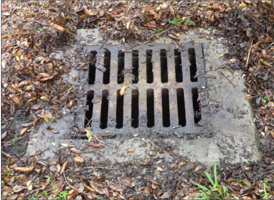
Stormwater Drainage Yard Inlet
