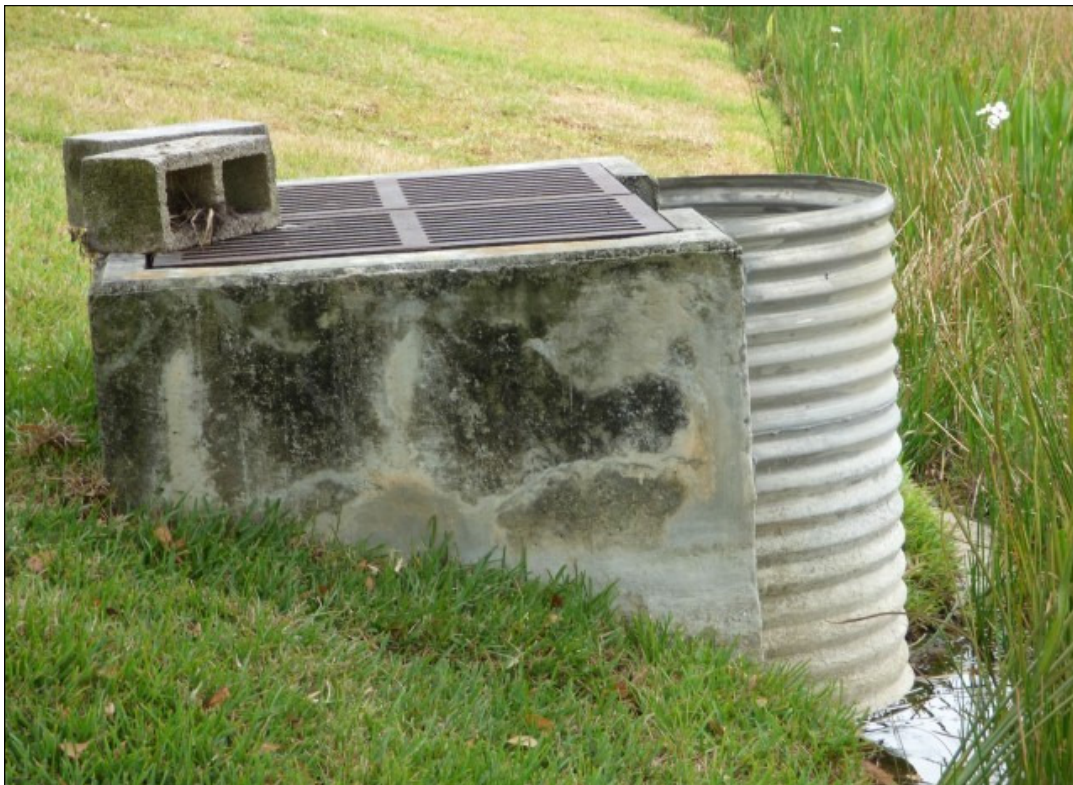
Stormwater Drainage Control Structure
