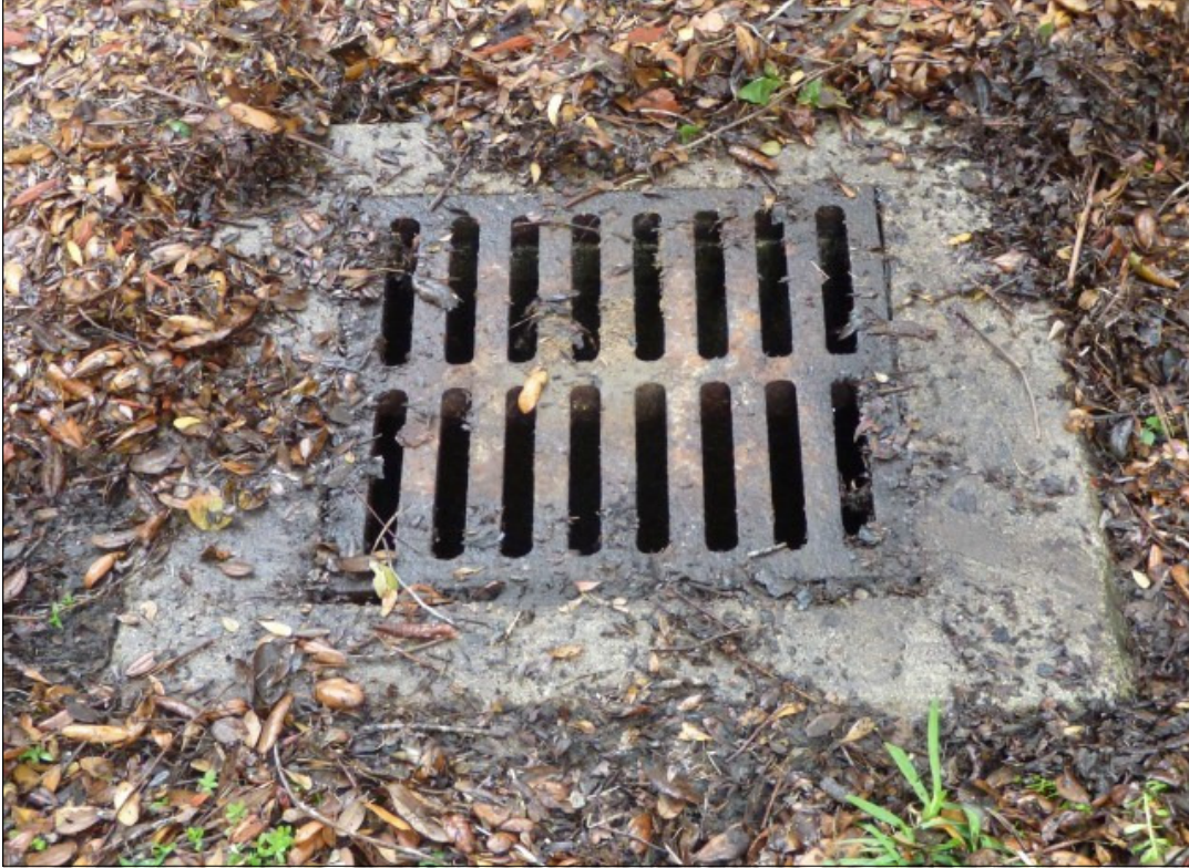
Stormwater Drainage Yard Inlet
