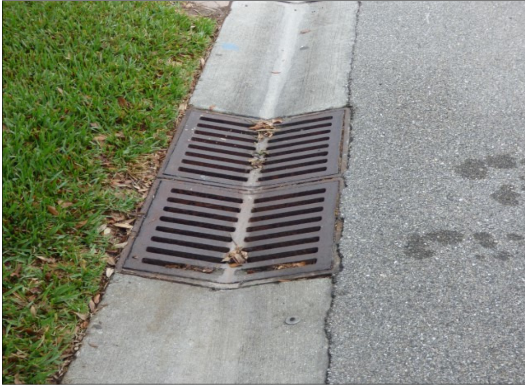
Stormwater Drainage Valley Gutter Inlet
